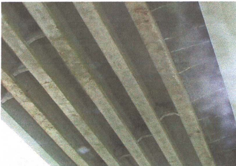
BOTTOM OF DECK
