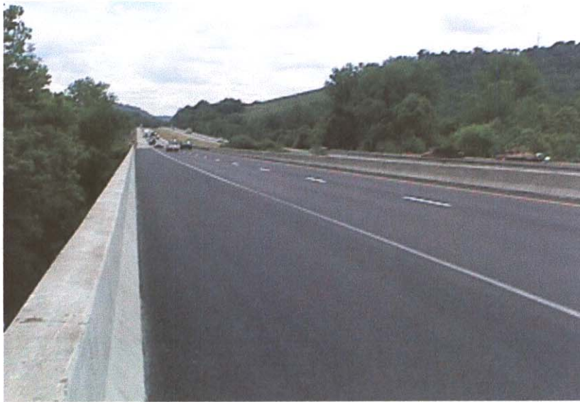
ACROSS TOP OF DECK
